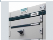
Standardized labelling system for sections and feeders
